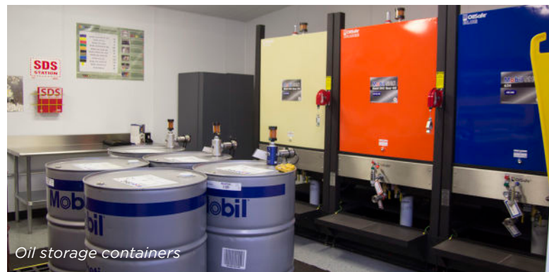
Top-up containers and grease gun storage
